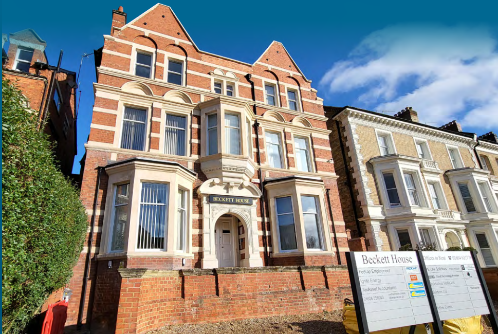
BECKETT HOUSE, 14 BILLING ROAD, NORTHAMPTON, NN1 5AW
